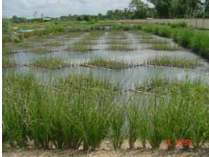
Photo 2: Vetiver floating pontoons on a pig farm in Vietnam
