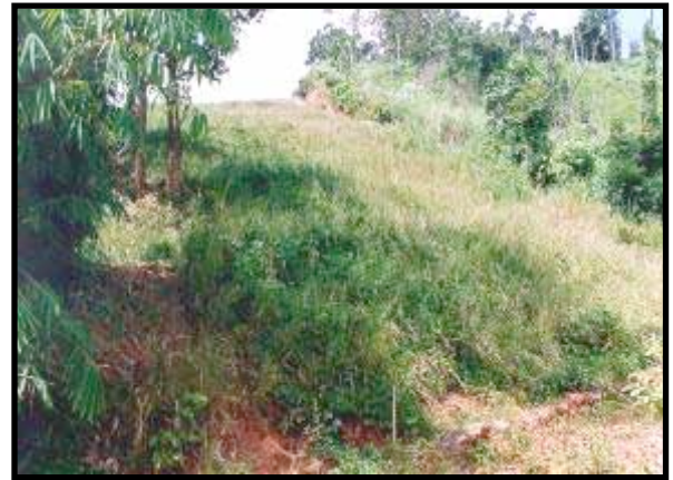
Figure 3. After rehabilitated by vetiver cultivating at KP12+300 in 1999.
