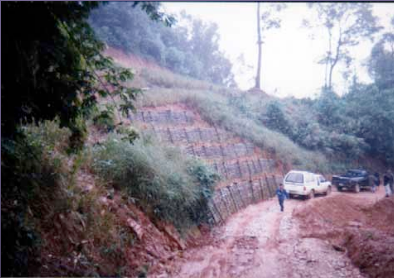
Figure 15: Control of soil erosion with vetiver technology on cut slope above the gas pipeline right of way in Kanchanaburi Thailand( PPT. :Photo)
