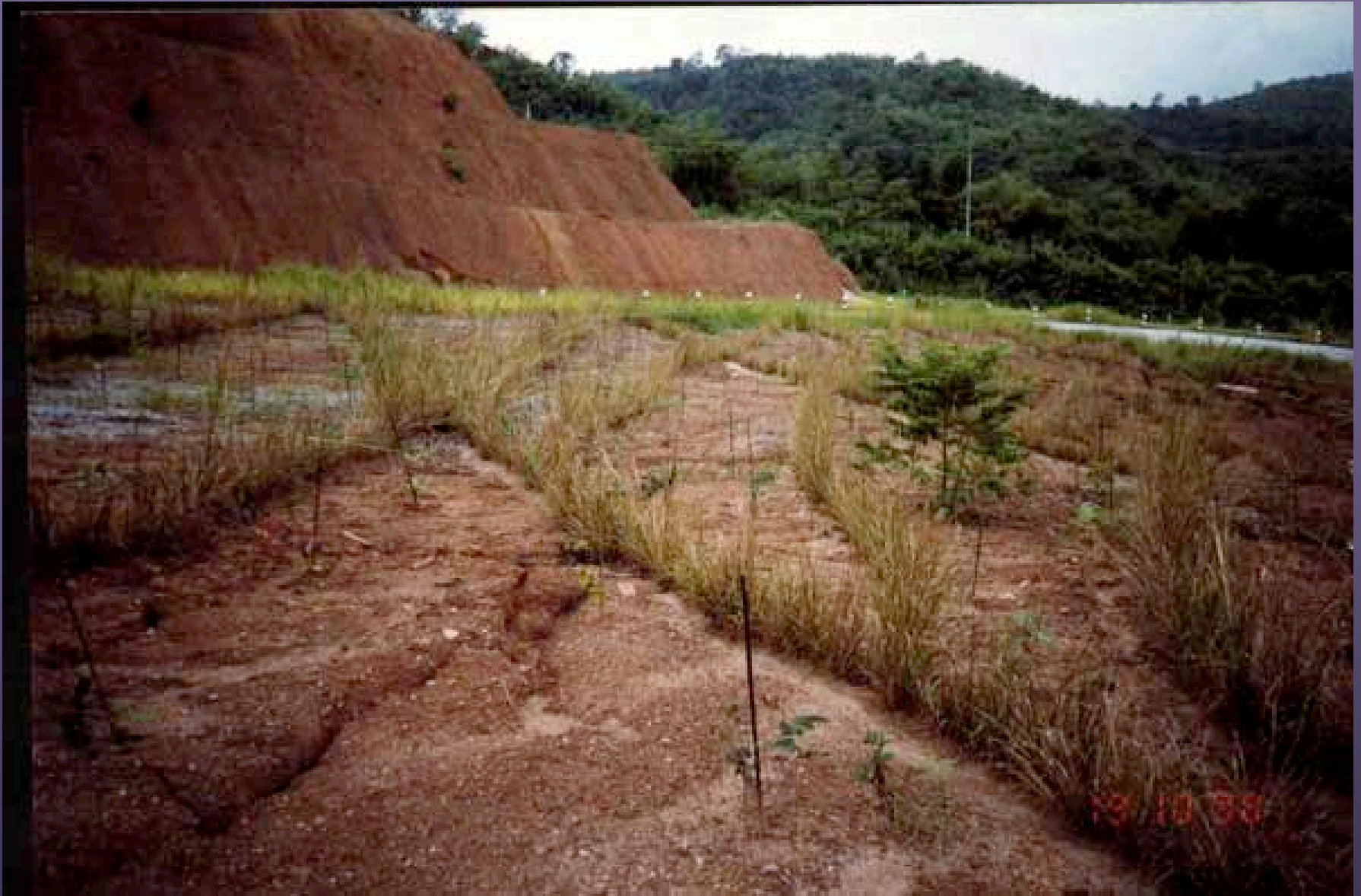
Figure 5. Well-established vetiver hedgerows network 6 month old to protect the ridges above the gullies and to diffuse run-off water.
