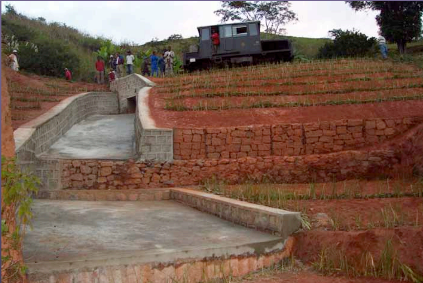
Figure 24: A restored cement drainage and vetiver hedgerows on the ground above railway Madagascar after cyclone damage (Hengchaovanich and Freudenberg : Photo)
