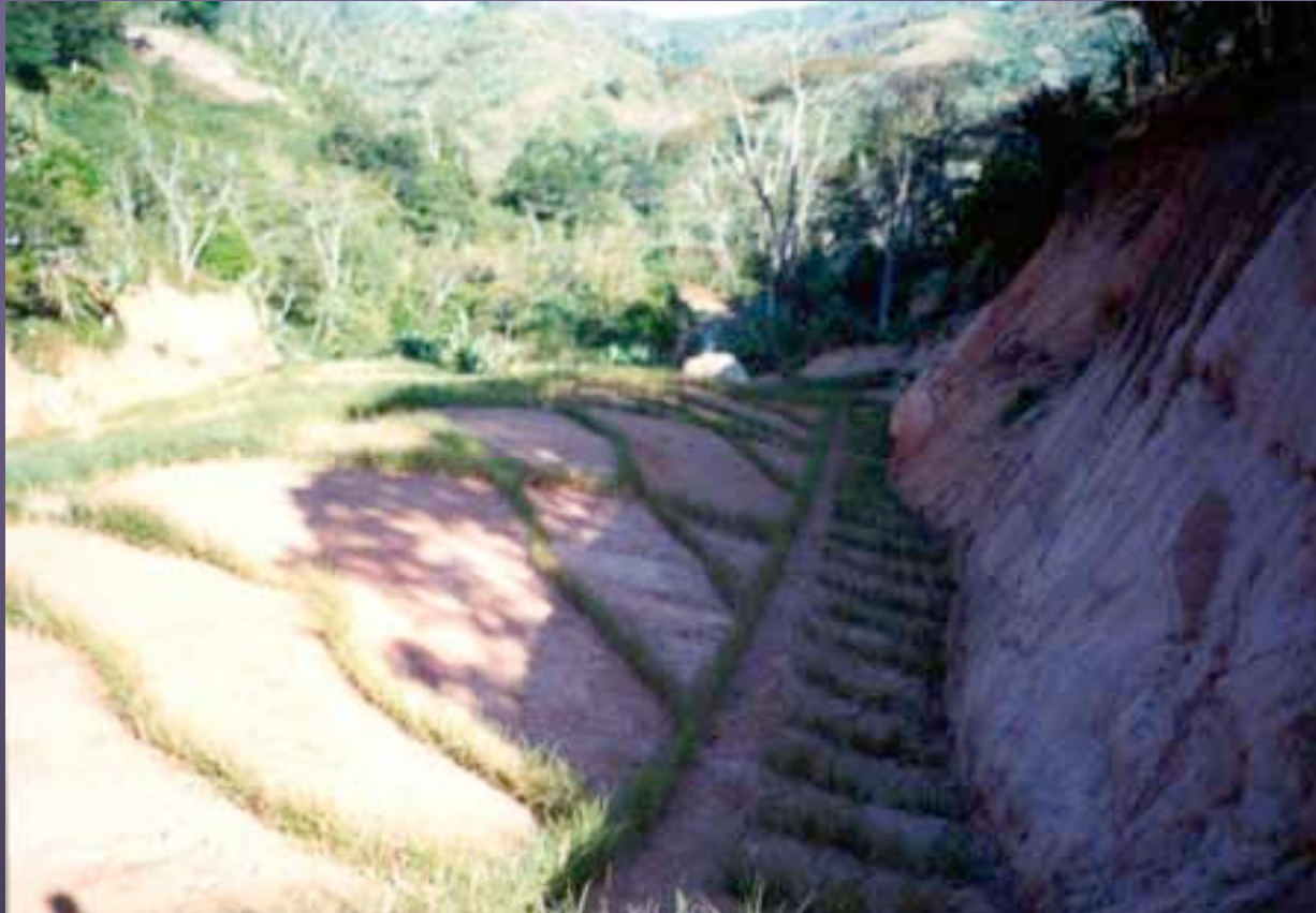
Figure 23 : Repair ground above railway tunnel in Madagascar after cyclone damage (Hengchaovanich and Freudenberger : Photo)
