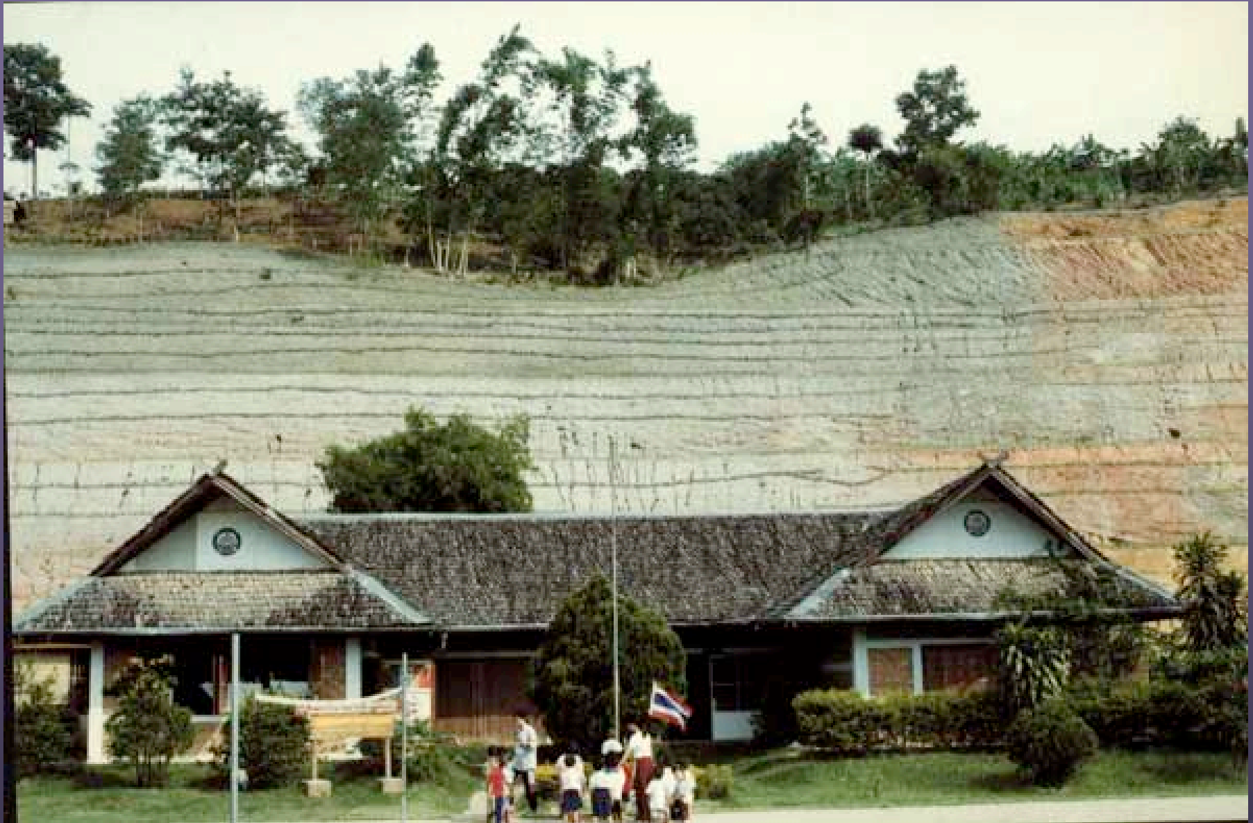
Figure 9: The same site as in figure 8 after making the terraces, planting vetiver hedgerows and hydroseeding of bermuda grass on the backslope.
