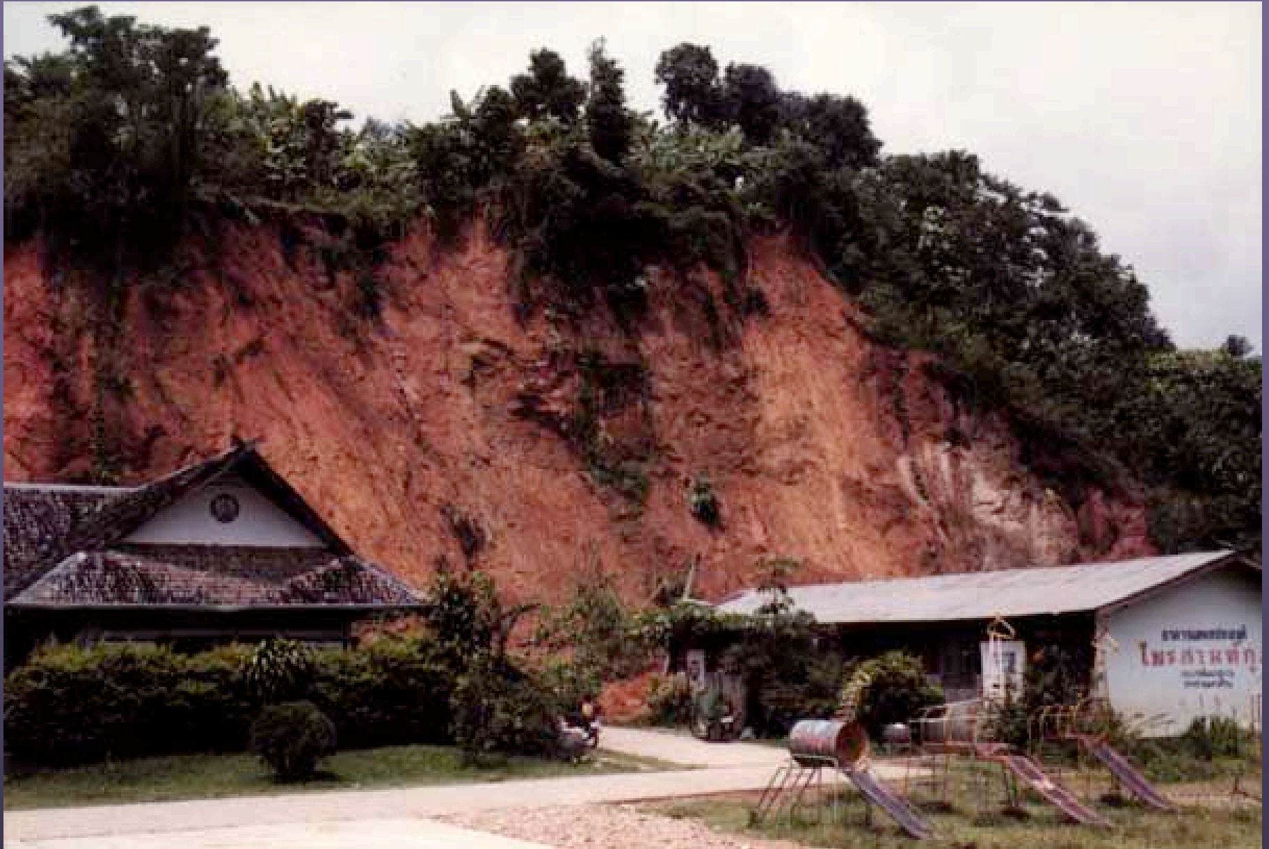
Figure 8. Landslide causing damages to the nursery and daycare center at Hauy Nam Kun village.
