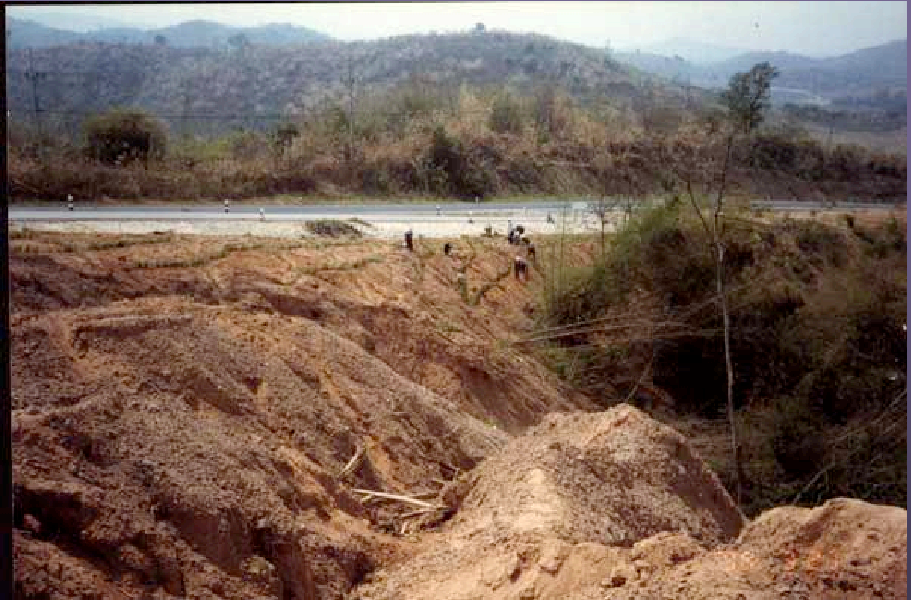
Figure 4 : Planting vetiver hedgerows to stabilize gullies on the road sideslopes.
