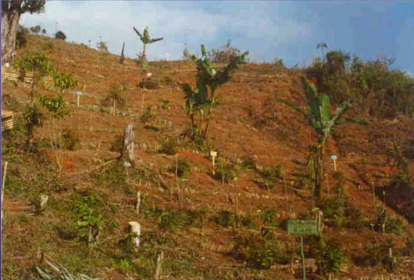
Figure 25: Vetiver technology in agriculture system on railway right of way (Hengchaovanich and Freudenberger : Photo)
