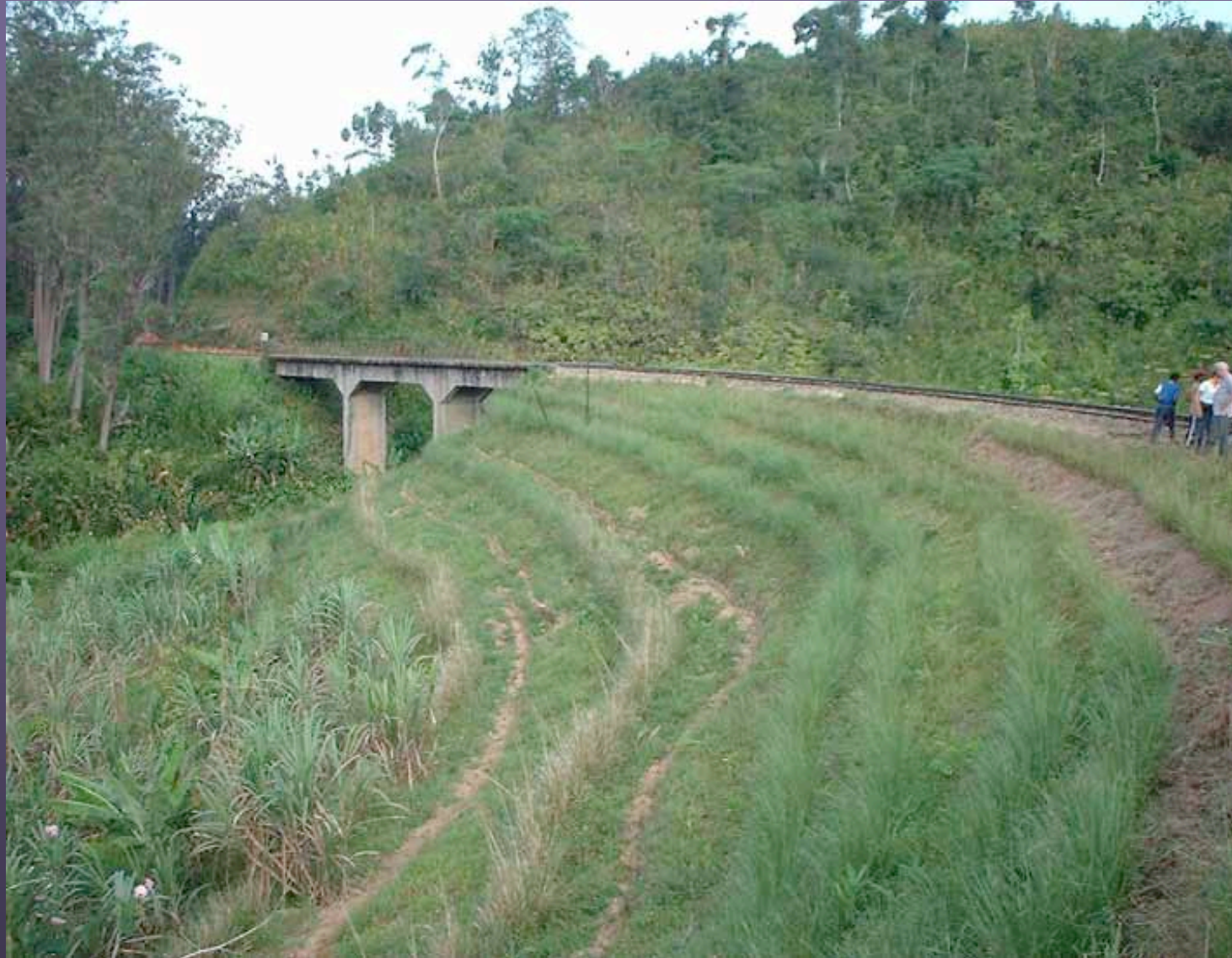
Figure 22: Restoration of railway in Madagascar after cyclone damage (Hengchaovanich and Freudenberger : Photo)
