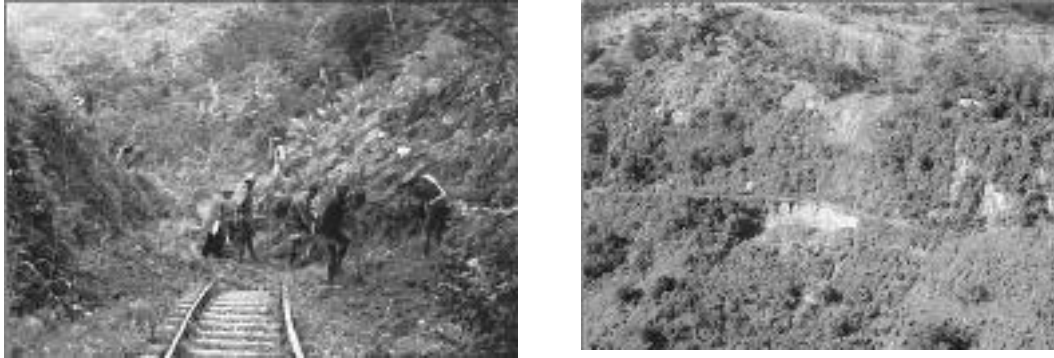
Fig. 2 Examples of devastating damage, Left , 280 landslides and Right , 28 embankment slides.
