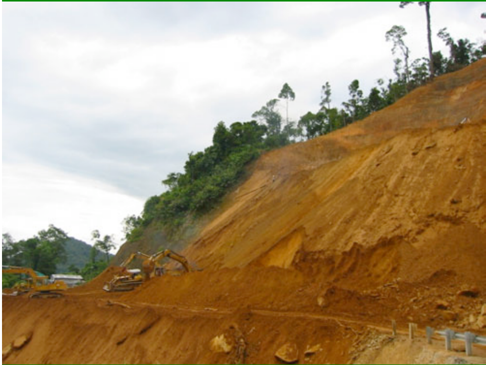
Above: A big landslide in the completely weathered granite at A Roang Pass, Ho Chi Minh Highway (Thua Thien-Hue province).
