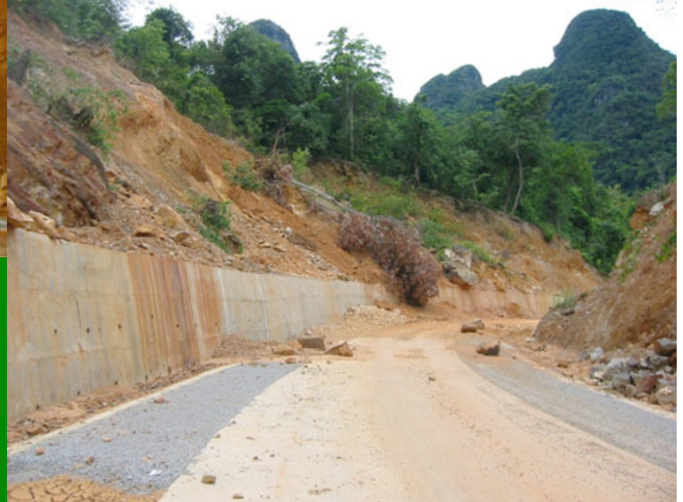
Below: Even a rigid concrete retaining wall did not help - a rock slide near Phong Nha (Quang Binh province).
