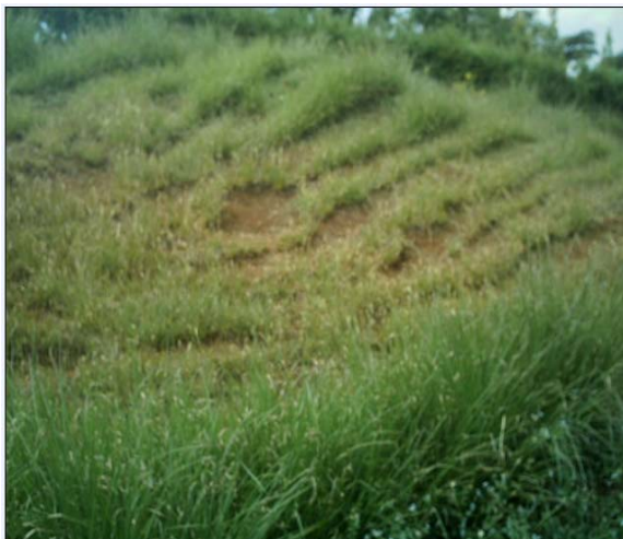
Fig. 7. Vetiver hedge rows used to stabilize the fill up/ cut soil at pulping stations in CPDE.
