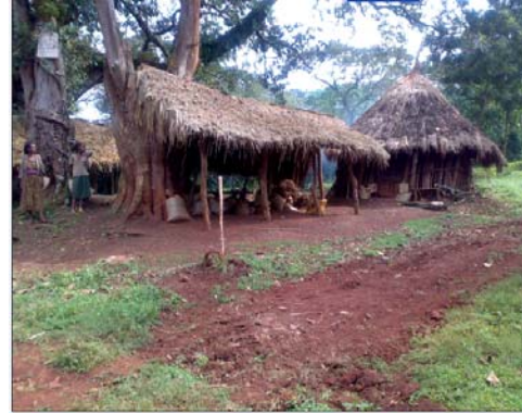
Fig. 10 Thatched shed using vetiver grass
