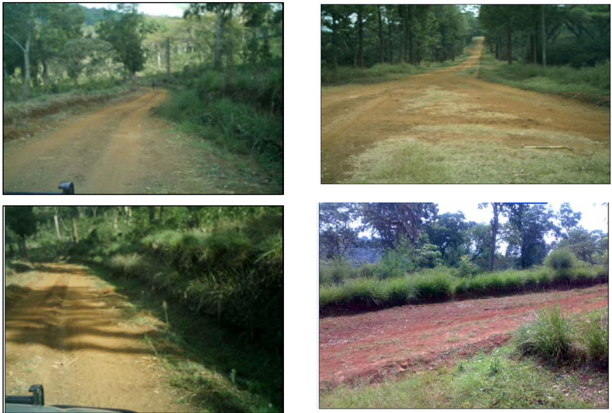
Fig. 6. Vetiver used to stabilize road verges at CPDE
