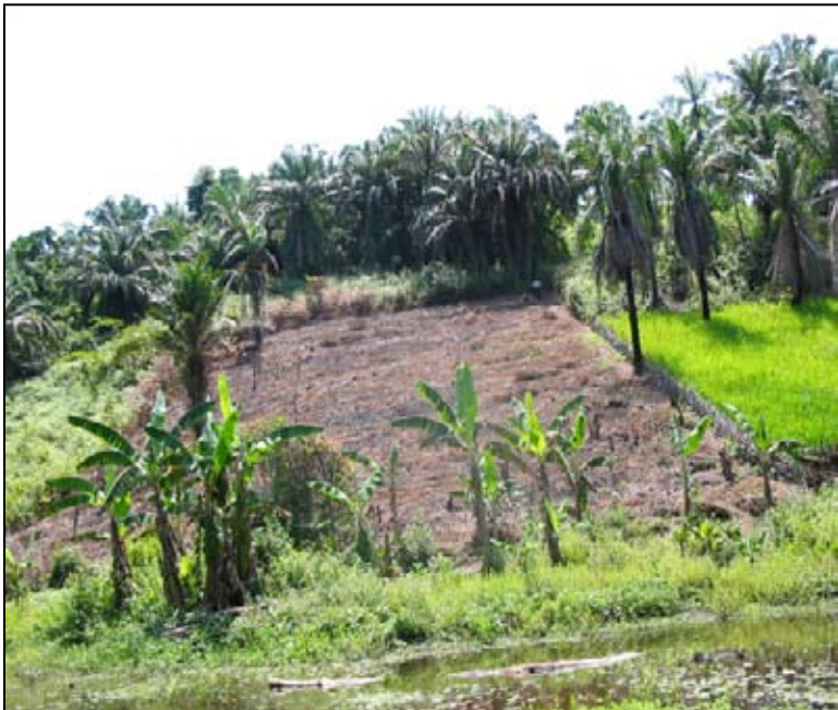
Photo 1: Typical unprotected and eroding slope
