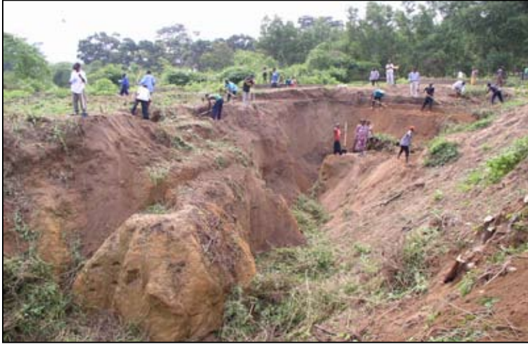
Photo 9: The problem - massive gully erosion.
