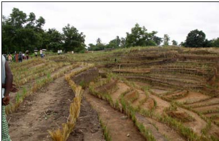
Photo 10: Reshaped gully with newly planted vetiver.
