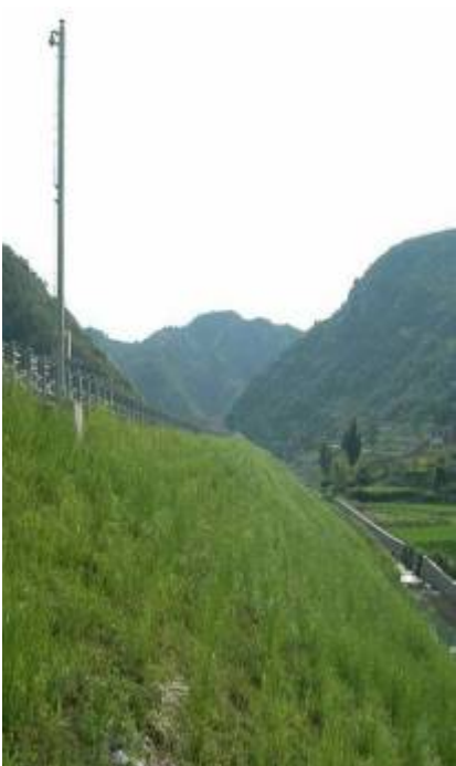
Photo 23 Vetiver protect highway.
