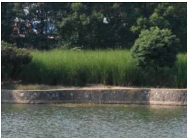
Photo 3. Using vetiver to protect water pool.
