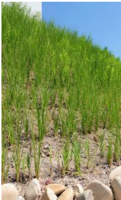
Photo 24 Slope protected by vetiver.
