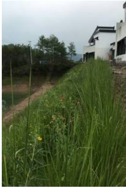
Photo 21-22 Vetiver to protect slope and houses.
