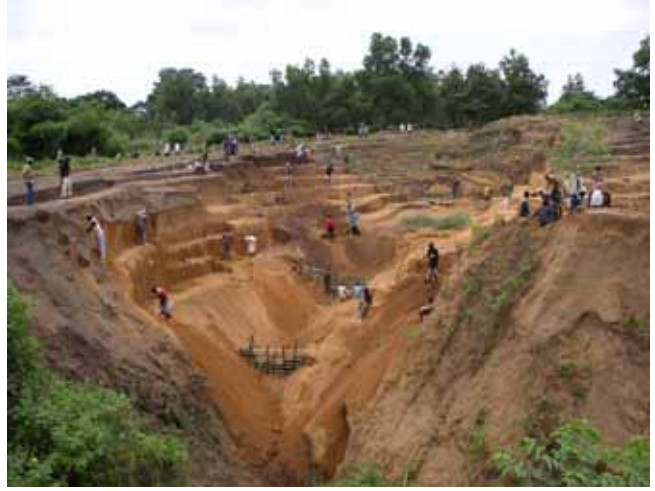
Re-profiling the ITPKA ravine slopes
