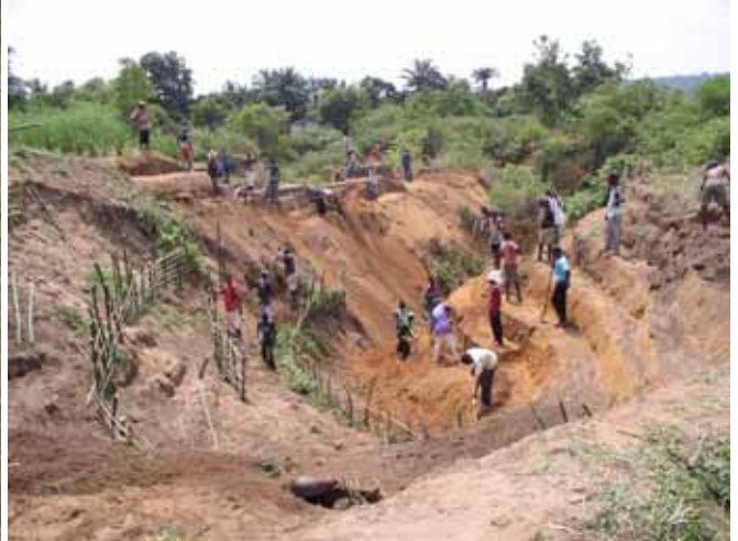
Retaining barriers built with tree branches providing temporary support for bench terraces on very steep and highly fragile soils
