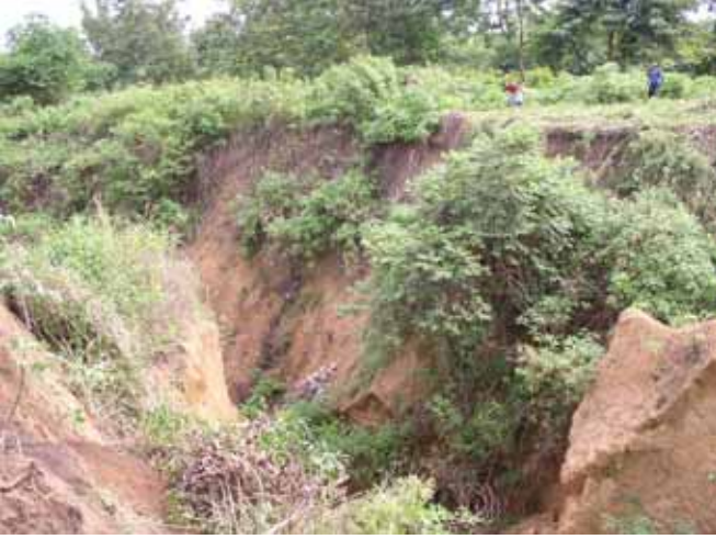
ITPKA Ravine before re-profiling
