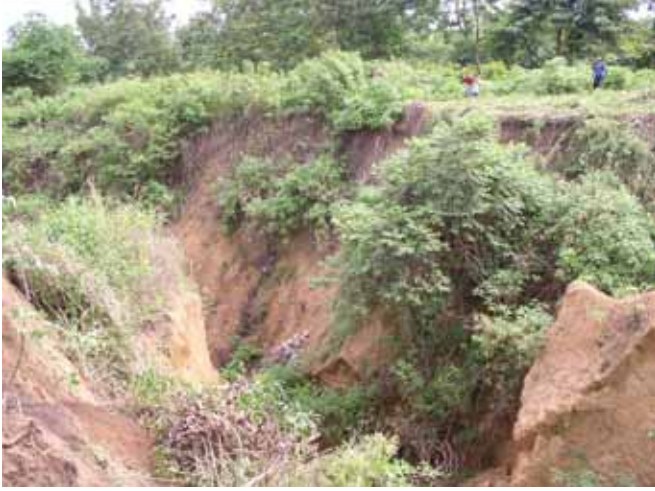
ITPKA Ravine before re-profiling
