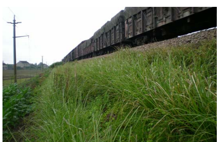
Railway was fully protected (7 years later after planting)
