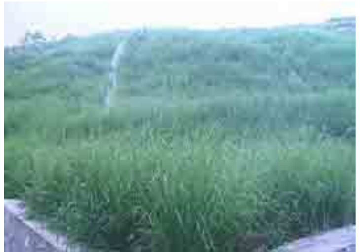
Huge highway cut was fixed by vetiver (elephant grass failed before)
