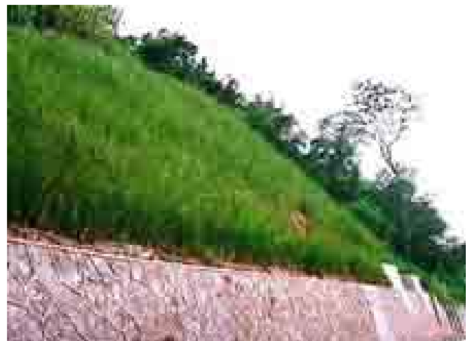
Slope stabilization (above and opposite are all buildings)
