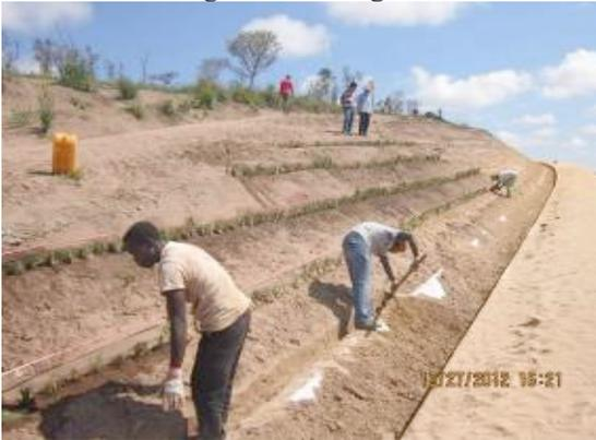
Photo 18, 19 Slope stabilization of National Highway No. 1, the Republic of Congo
