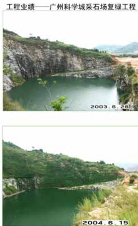
Fig. 30 Up: the original whole appearance of Lichi Hill Quarry before revegetation. Please note the huge water pit quarried Down: the rehabilitated whole appearance 8 months after the revegetation project was over
