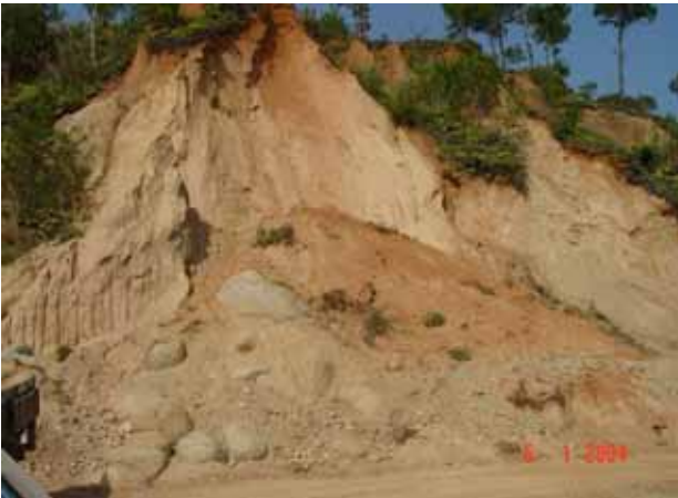
Fig. 23 Another slope of the reservoir assuming severe landslide, which would also be reined with the vetiver eco-engineering
