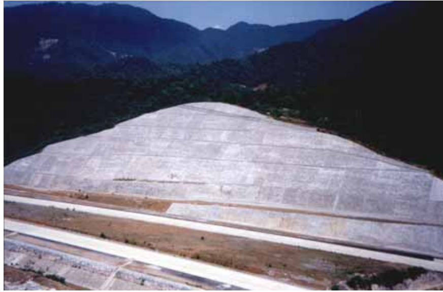
Fig. 11 A section of highway being constructed in northern hilly region of Guangdong The huge up-slope is covered by cement wall that is very expensive and short of ecologic benefit
