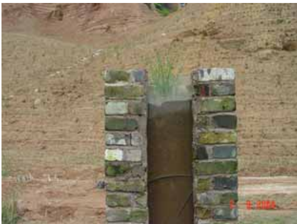
Fig. 28 An observation box for investigating growth of vetiver roots was set up on the spot on August 25 th , 2004
