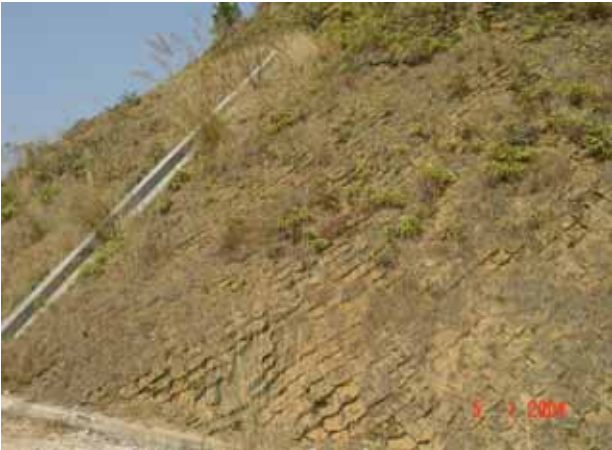
Fig. 21 A failed project of planting grass in lattices set on a slope of the reservoir conducted several years ago
