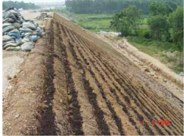
Fig. 13 A section of slope on the Zhangjiang section of Zhangjiang-Chongqing highway that is ready, dug up and manured, to be planted with vetiver
