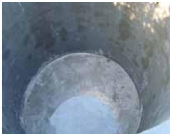
A new pond finished
