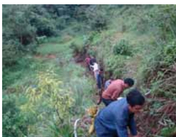
Install water pipes
